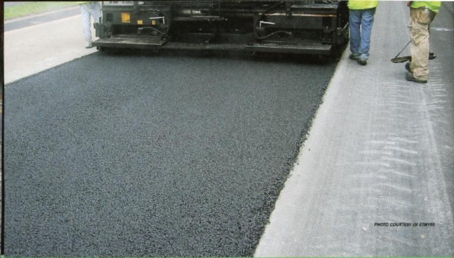
Placing an ultra-thin bonded wearing course
