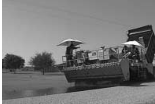
Chip sealing protects new pavements, increases macrotexture, and prolongs the life of structurally sound pavements that show surface distress.
