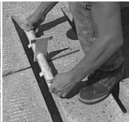
Load transfer restoration on portland cement concrete pavement: (left) cutting a slot in the pavement; (right) inserting dowel.
