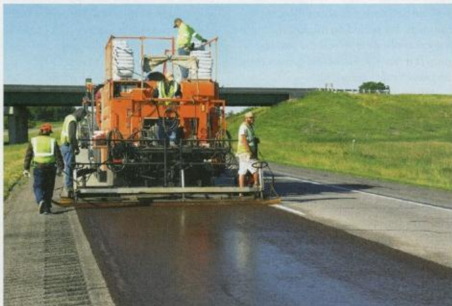
That microsurfacing can be used for both high-level interstate pavements as well as residential streets is a testament to their utility. Microsurfacing mixes are engineered products that use high-performance materials. Photo courtesy of BASF Corp.
